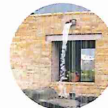
Wall sculpture: water discharges from stormwater detention chamber under parking through sculpture in retaining wall to vegetation below.
